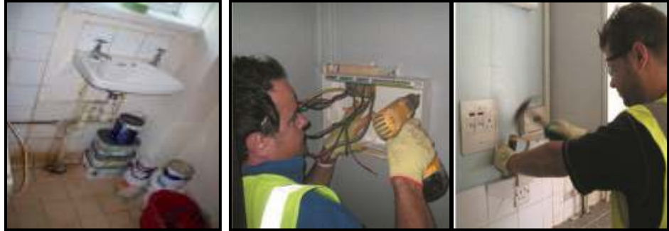
Bathroom Removal Electric Rewire Plastering / Patch
