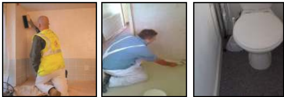
Tiling Decoration Floor Laying
